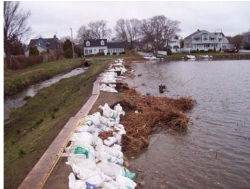
Sand Bags Protect the West Embankment at Easton's Pond
